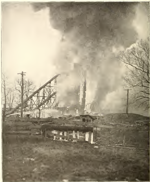
A BLENDING-TOWER FIRE. THE FLARE-UP CAUSED BY THE EXPLOSION OF FIFTY TONS OF SMOKELESS POWDER AT ONE OF THE WORKS OF E. I. DU PONT DE NEMOURS & CO.
